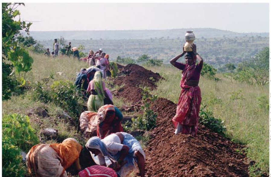
Women in India carve terraces to help in the capture of rainwater.
